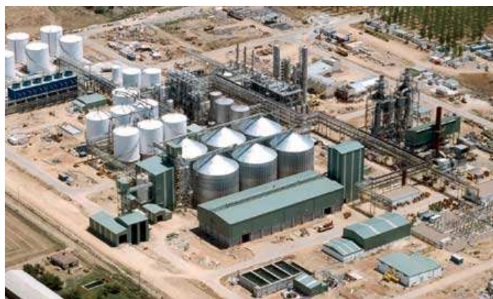
Figure 15. The bioethanol plant in Salamanca [5].
